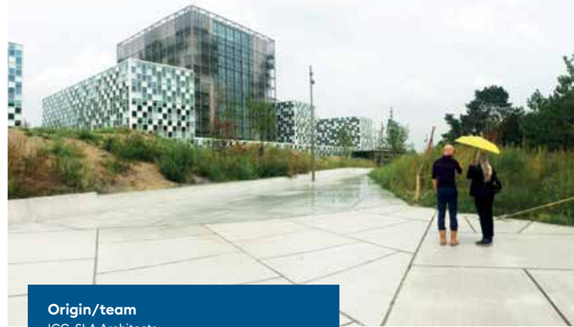
Photo: SLA Architects
